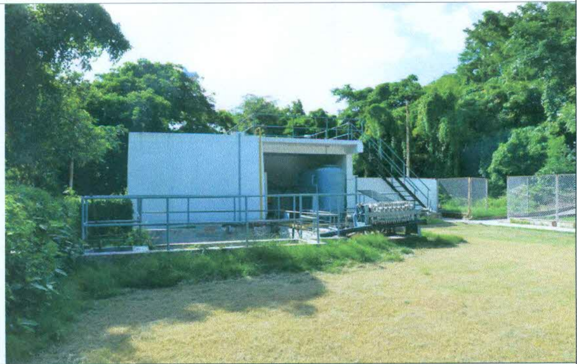
SEWAGE TREATMENT PLANT
