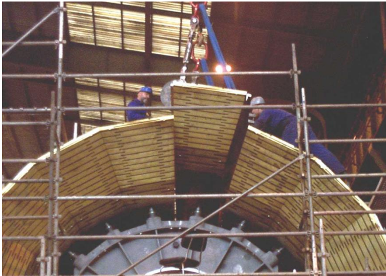
Scintillator Tile Assy. for Outer Hadron (HO) Calorimeter of CMS Expt. (Slided Partial View).
